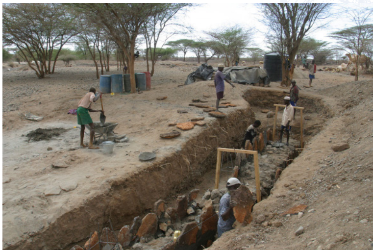
Setting up a sand dam
