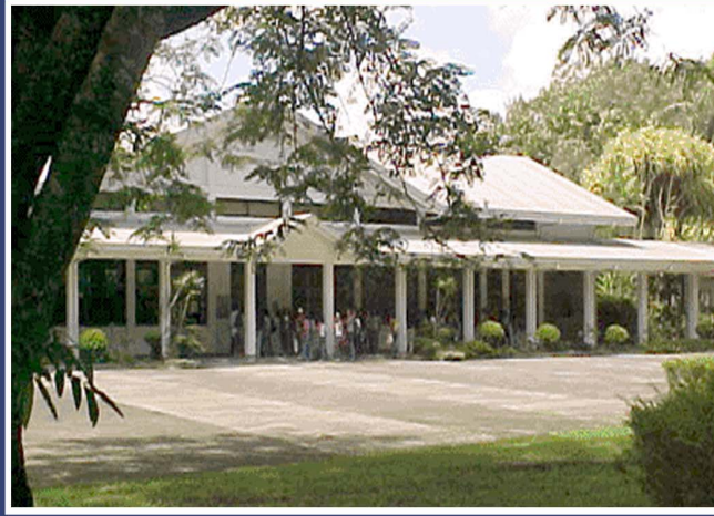
The Y.C. James Yen Center in Silang, Cavite, the Philippines serves as a training, workshop and conference facility for development practitioners from around the world and houses IIRR's Headquarters and Regional Center for Asia.
