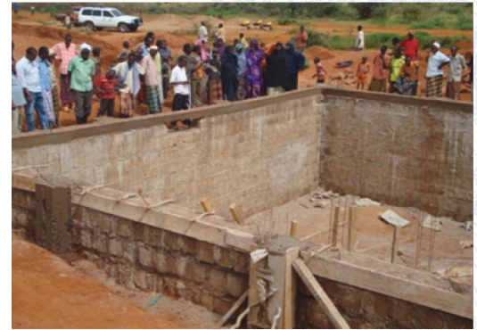
An underground tank under construction
