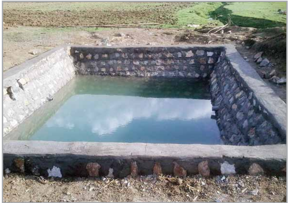
Construction of water harvesting structures.
