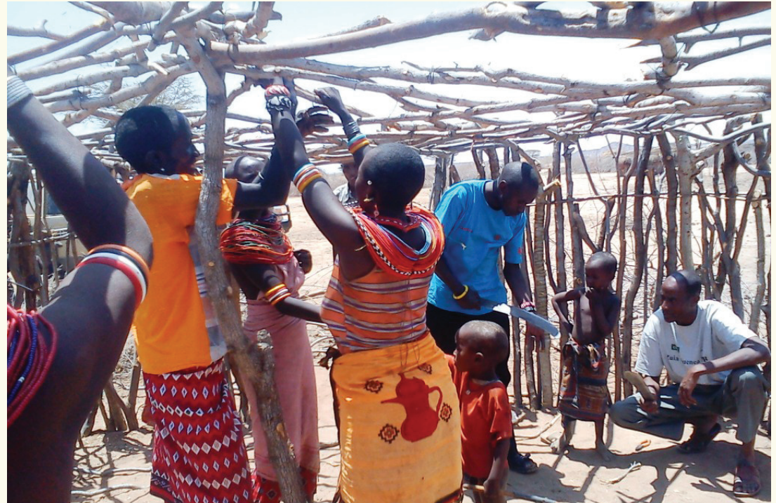
Parents constructing a learning shed.
